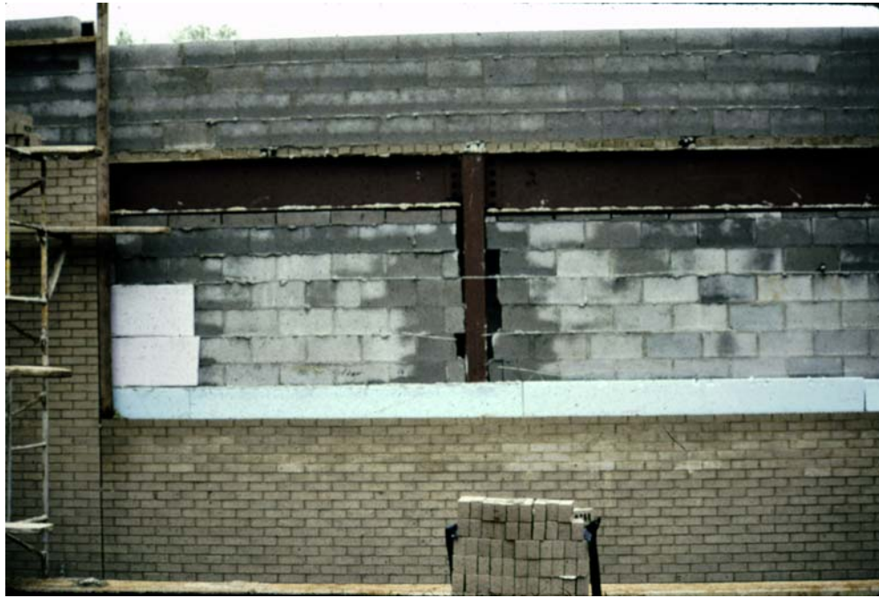
Photograph 6: Note absence of drainage plane – problem in the making
