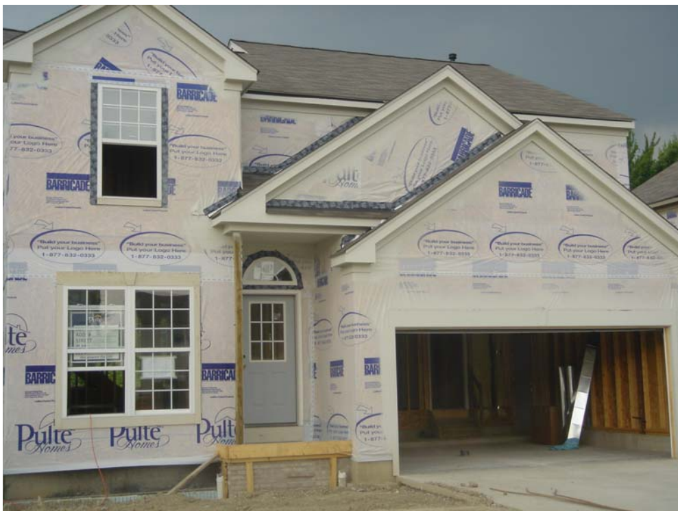
Photograph 2: "Housewrap" drainage plane
