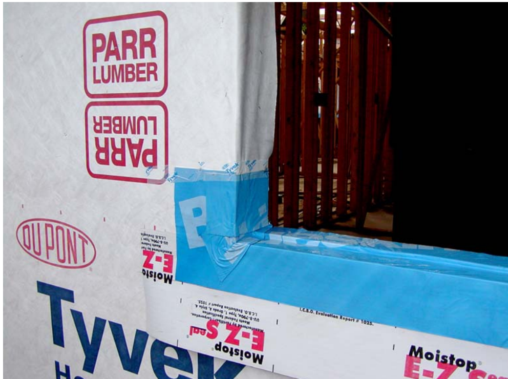
Photograph 7: Membrane lining window opening creating a "pan flashing"
