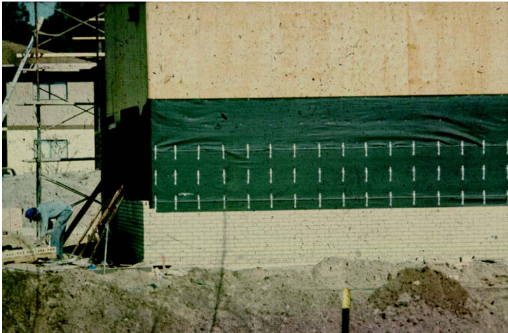
Photograph 1: Tar paper or building paper drainage plane
