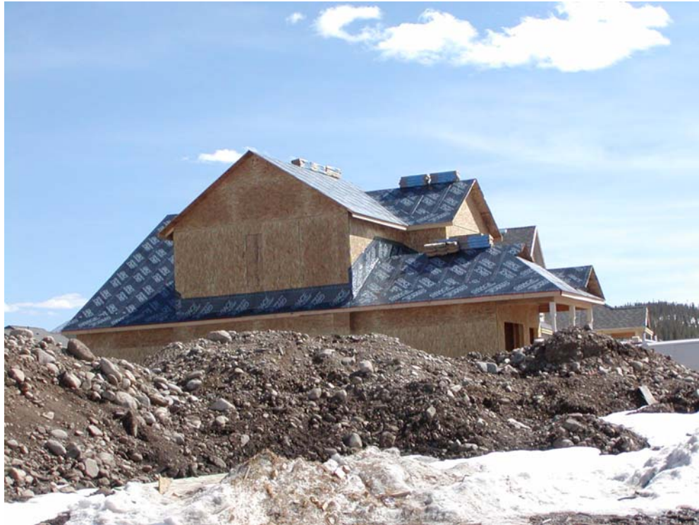
Photograph 8: Membrane connecting dormer drainage plane to roof drainage plane
