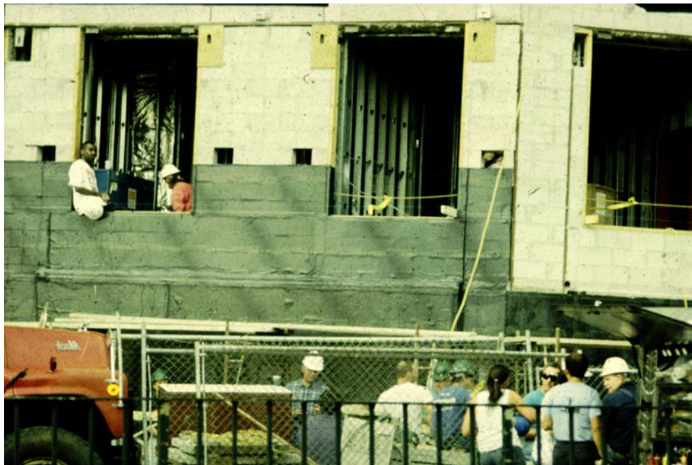
Photograph 4: Fully adhered sheet membrane drainage plane (and "air barrier" and "vapor barrier")
