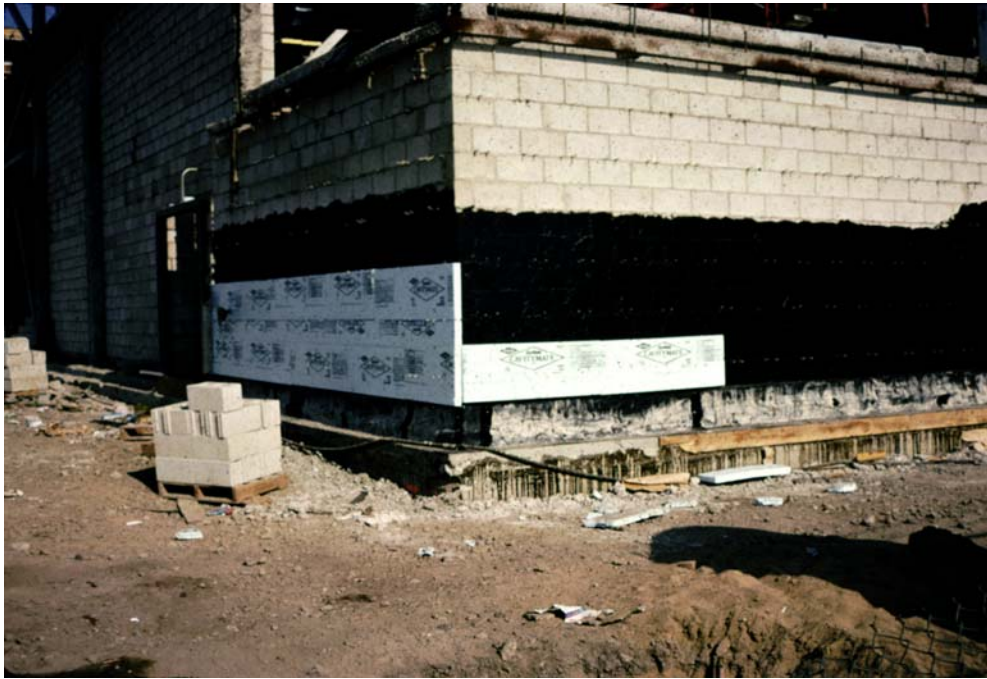
Photograph 5: "Trowel-on" drainage plane
