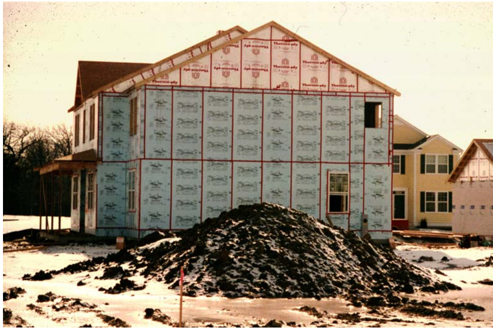
Photograph 3: Rigid foam insulating sheathing drainage plane
